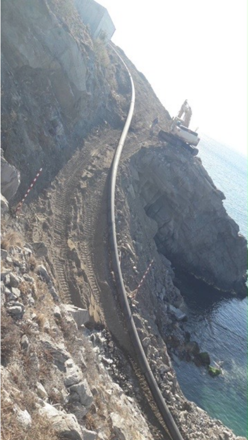
Submarine pipe for treated wastewater disposal
